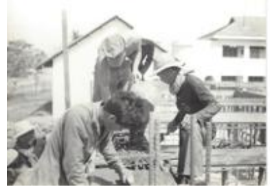
Team Member placing concrete with Vietnamese help
